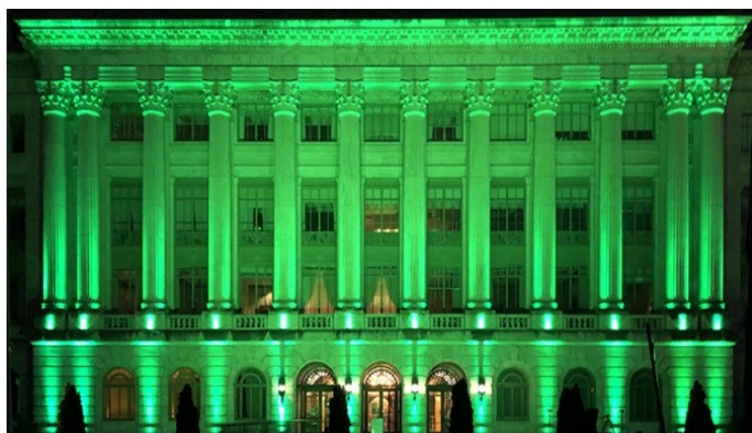
USDA Headquarters (Jamie L. Whitten building) on the National Mall in Washington DC. Photo by K. Cecilia Sequeira.
