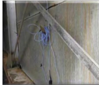
Sensors should consider the location of cold spots in the kiln (e.g. exit side of the air flow, etc.)
